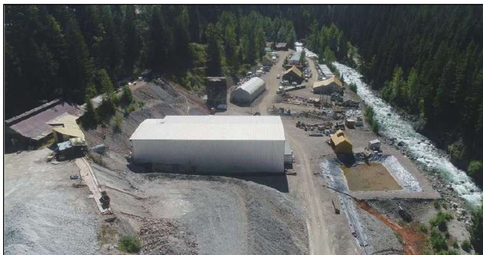
Bralorne Facilities Bralorne, BC, Canada
