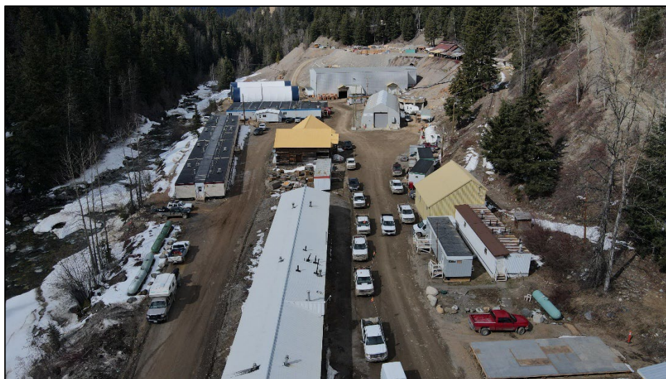
Bralorne Facilities Bralorne, BC, Canada
